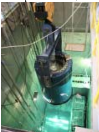
Figure 3: Loading under water and storage of the CASTOR BR3® cask (one can notice at the top of the casks, the connections for the pressure sensor)
